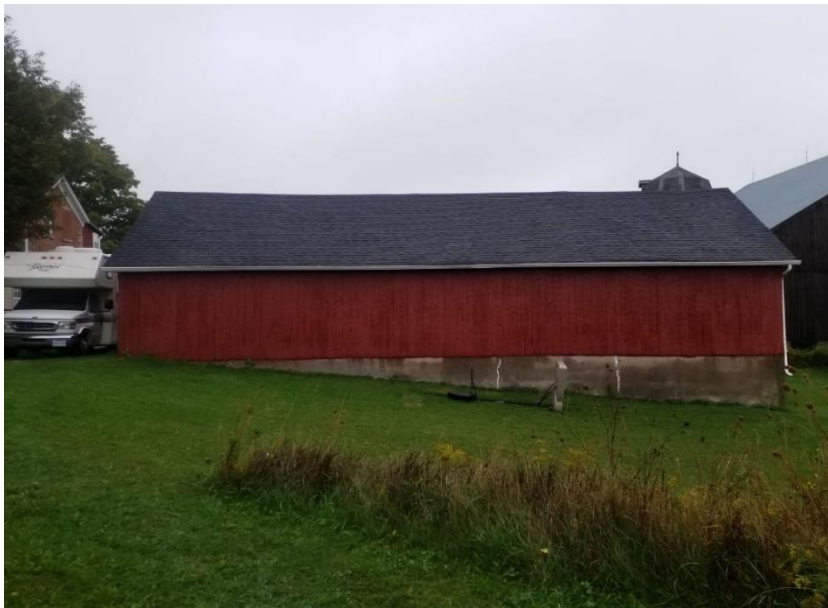
Image 2: View of barn within farm complex.
