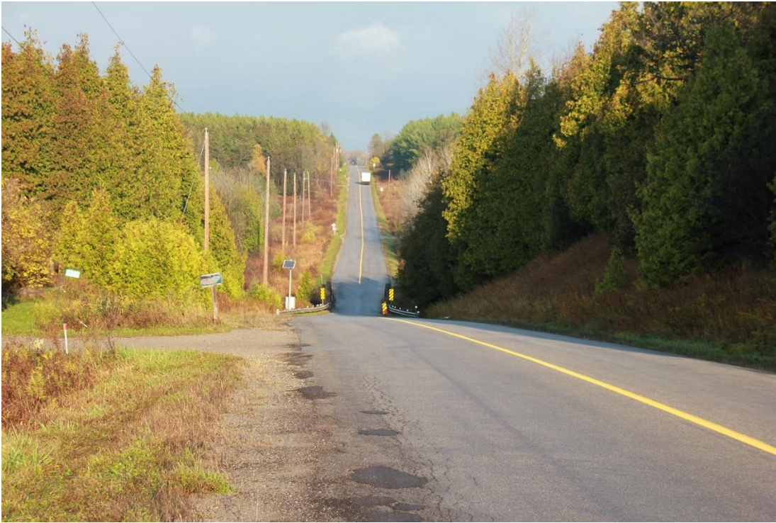
Figure 6 – 10 th Line West Credit River Bridge (CVC monitoring station also pictured)
