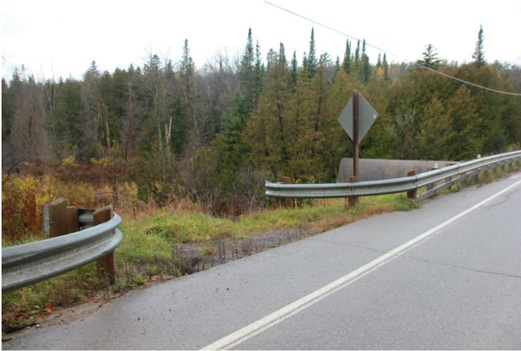
Figure 14 - West Side of Winston Churchill Blvd River Crossing
