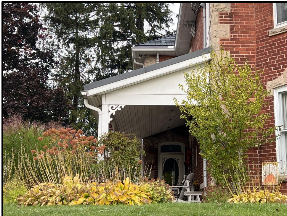
Image 4: Detail of Side Porch and Entranceway on West Elevation of 3 Station Street (Photo taken October 19, 2023; Facing Northwest)
