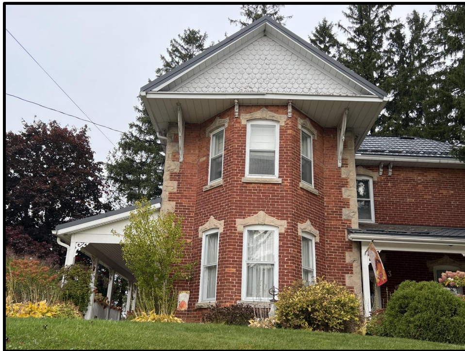
Image 2: Detail of Front Gable and Projecting Bay on Façade of 3 Station Street (Photo taken October 19, 2023; Facing Northwest)
