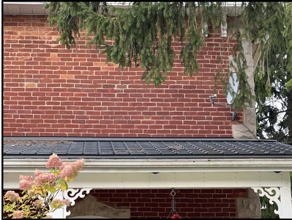
Image 5: Detail of Brick Bond and Stone Quoins of 3 Station Street (Photo taken on October 19, 2023; Facing Northwest)
