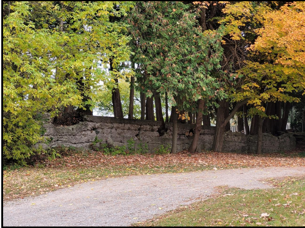
Image 9: Detailed View of Retaining Wall of 3 Station Street (Photo taken on October 19, 2023; Facing West)
