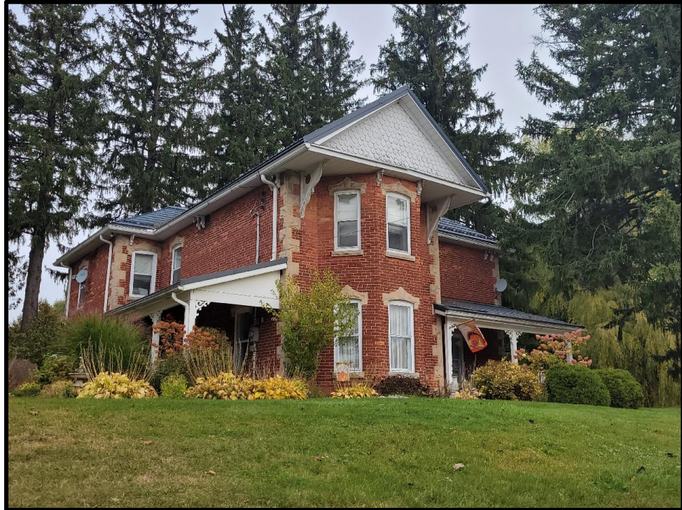
Image 10: South and West Elevation of 3 Station Street (Photo taken October 19, 2023; Facing Northwest)
