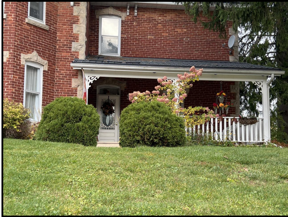
Image 3: Detail of Porch and Entranceway of 3 Station Street (Photo taken October 19, 2023; Facing Northwest)
